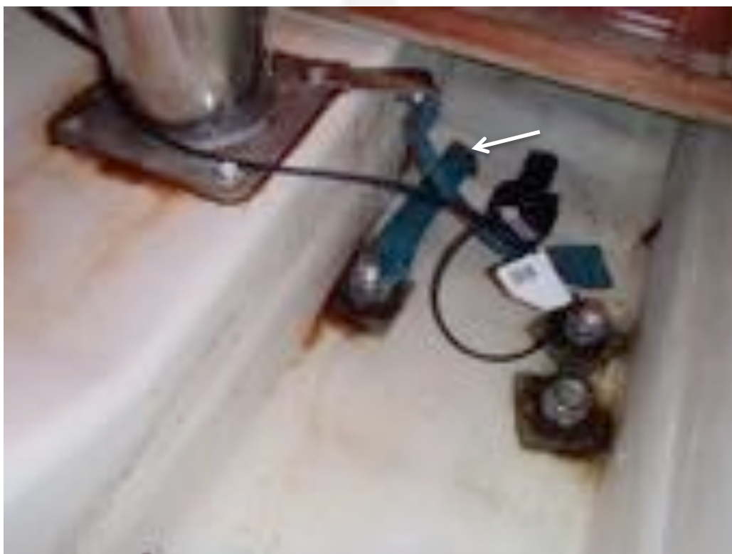
Image of the forward bilge. Note the base of the compression post and green corroded grounding strap which has parted.
