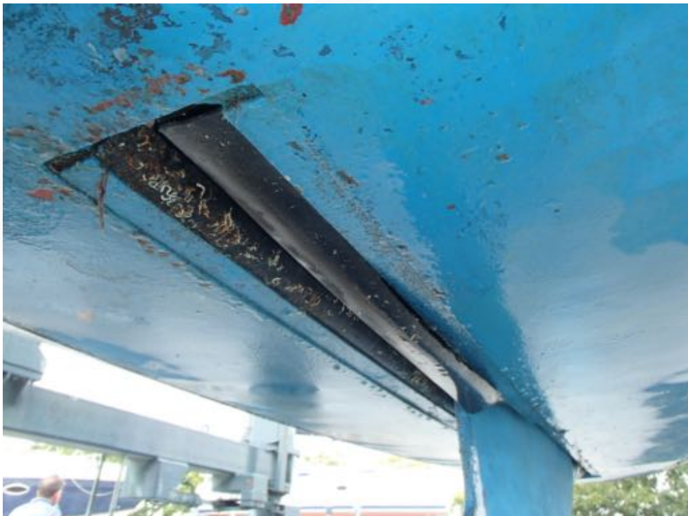
Image of the keel box aperture. Heavy fouling was noted around and inside, and the rubber collars either side were damaged
