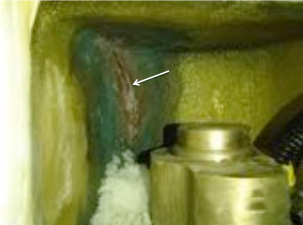
Image of the port stock and surrounding alloy cover. Note the weep form a suspected split in the cover.
