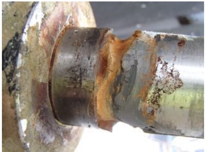
This is crevice corrosion at its very worst! This was a propeller shaft from a 5 year old vessel. The shaft alloy was sub-standard. This was a charter vessel and the corrosion was only picked up during my survey when the vessel was sold.
