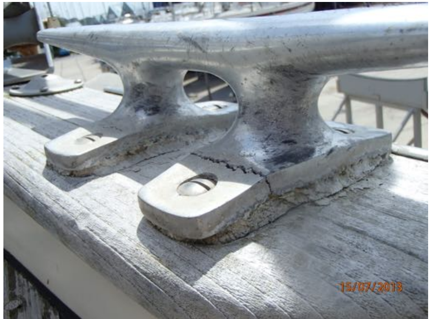
Image taken of a bow mooring cleat on a Hallberg Rassy. Stainless steel bolts, aluminum cleat and seawater all great ingredients for corrosion. Note the impressive crack on the foot of the cleat.
